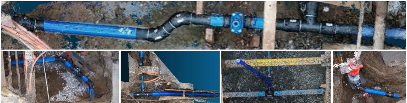
Fig. 3: 3D reconstructions of excavation sites from our data set, depicting the predominant use of straight pipes and T-junctions. When hard pipes are used for water or gas, they show only sharp angles of 45^\circ , 60^\circ , or 90^\circ , as shown in the bottom left image. Some reconstructions also show a small outgoing branch, as seen in the top image. Occasionally, pipes are partially covered by dirt, as shown in the bottom row, third image.
